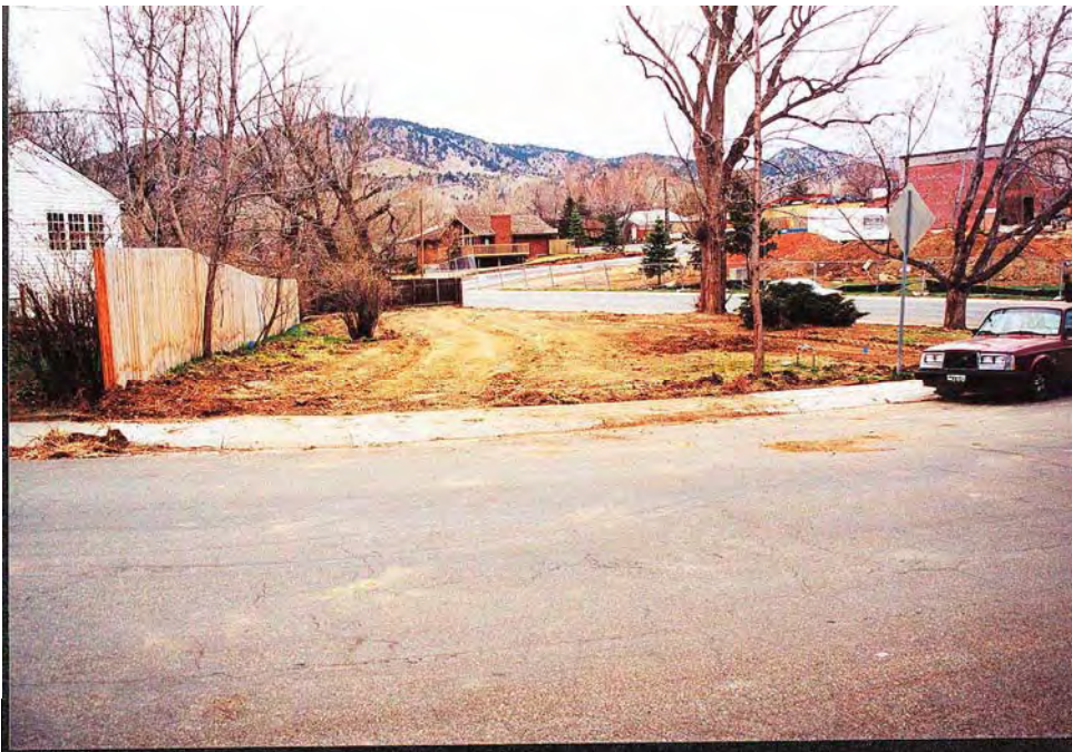
Photograph 3. Site preparation. No topsoil was added. End of March 2000.
