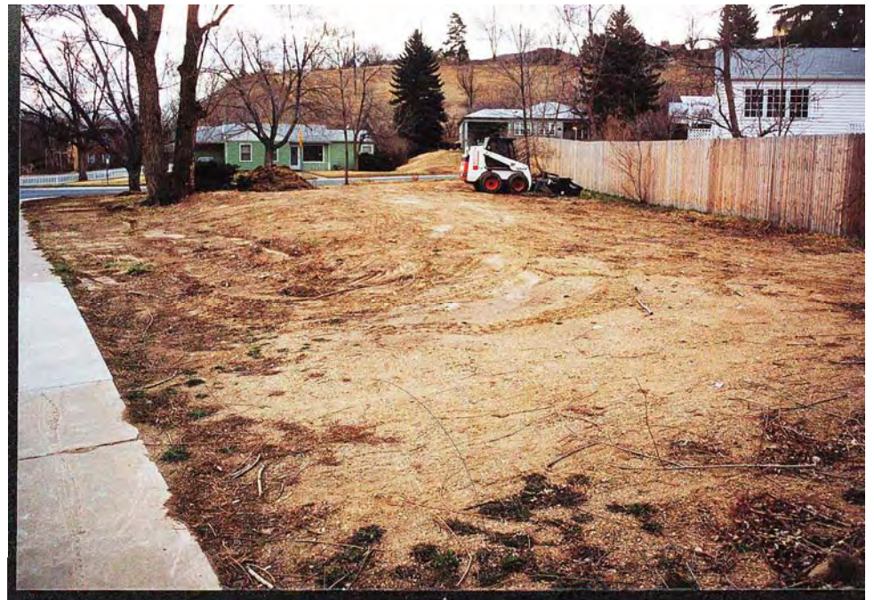
Photograph 4. Site preparation. No topsoil was added. End of March 2000.
