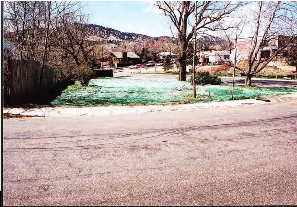
Photograph 5. After application of seed and hydraulic mulch. April 2000.
